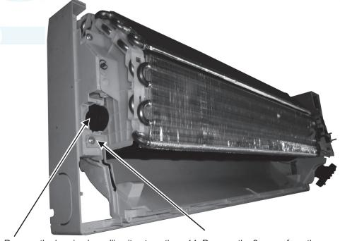
15 Remove the bearing by pulling it out gently. 14 Remove the 2 screw from the evaporator
