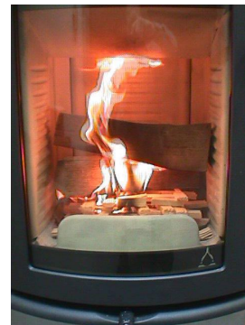
Figure 4: close the primary air
