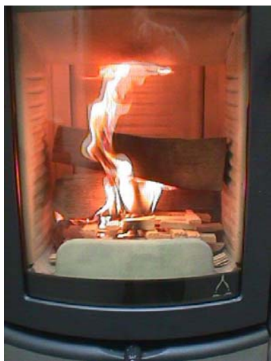
Figure 5: Close the Primary Air
