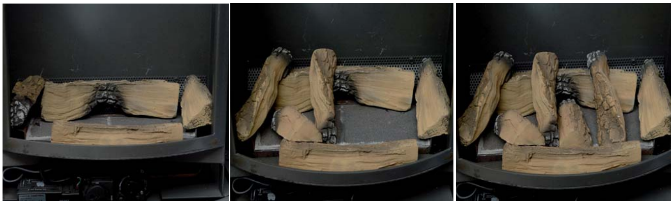
Arranging the log set for natural gas
